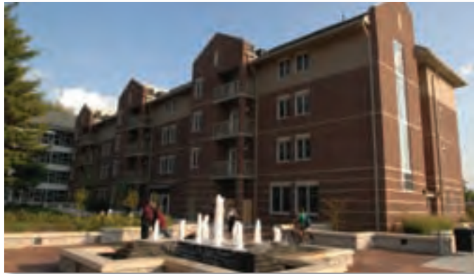
Figure 2-9. New student apartments at Wall and Grand Streets.
